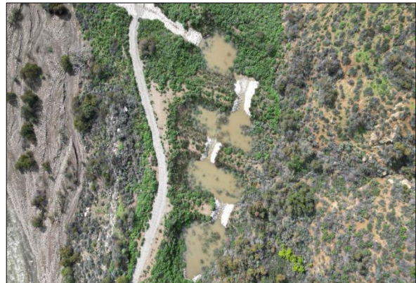
Figure 3: Settling Ponds (January 16, 2023) Source: Report of Operations – January 2023 San Antonio Creek Spreading Grounds Project Pilot Diversion Test (February 21, 2023)
