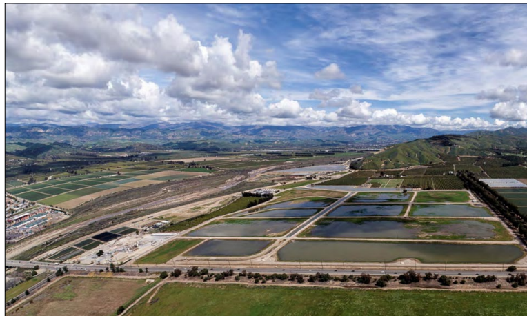
Figure 9: Saticoy Groundwater Recharge Facility Source: United Water Conservation District
