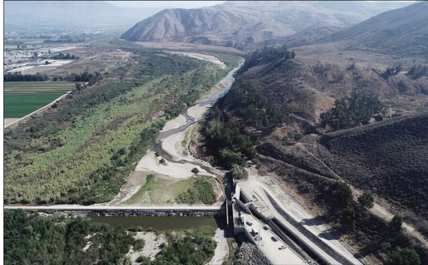
Figure 8: Freeman Diversion Source: United Water Conservation District
